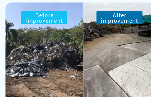
▲ Require suppliers to improve their operating environment
